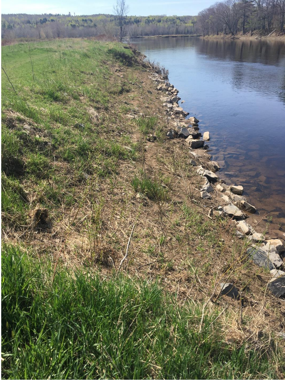
B03b. NWAI bank stabilization project. Photo taken post-flooding on May 21, 2020 at 10:40am.
