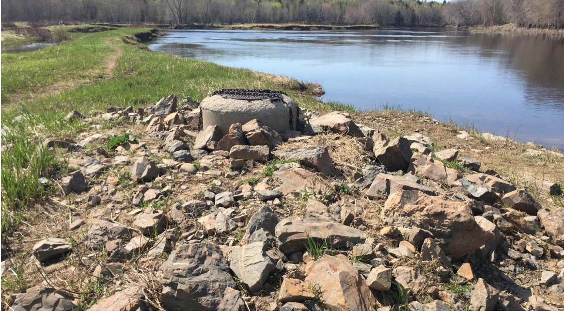
B04a. Storm drain. Photo taken on May 21, 2020 at 10:46pm.
