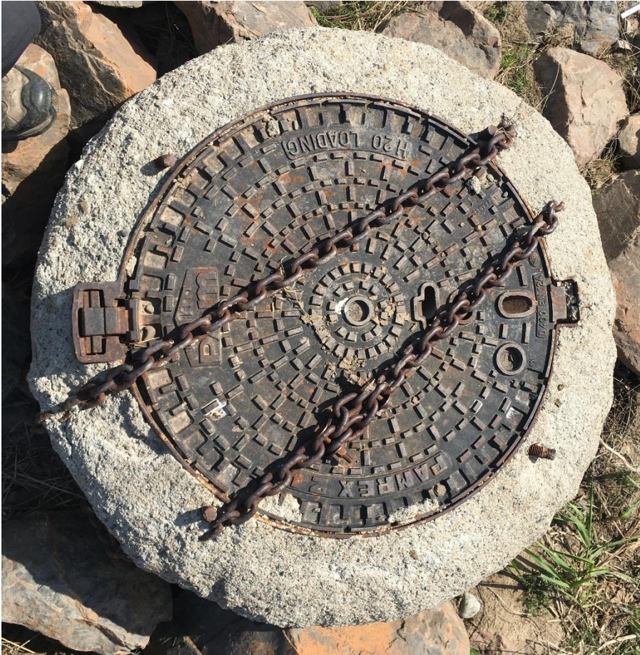
B04b. Storm drain. Photo taken on May 21, 2020 at 10:46pm.
