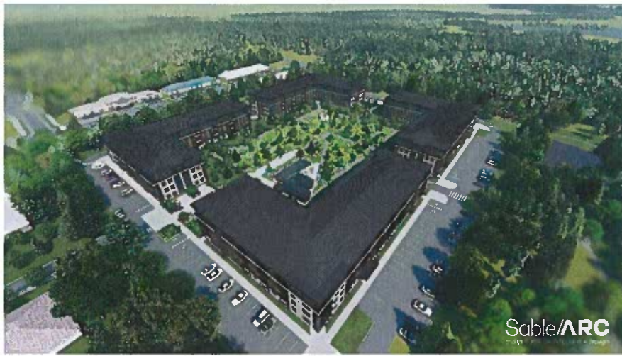
Northwest / Nord - Ouest
