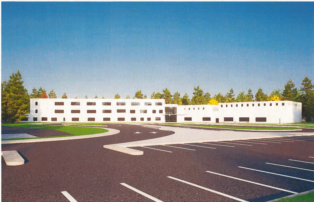
Front (North) / Façade (Nord)
